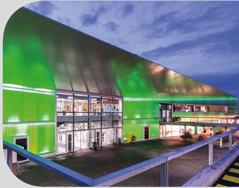
Migros shopping centre, Romanel, Switzerland
