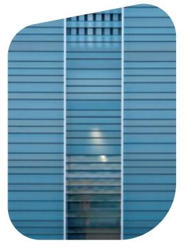
Installed horizontally: the façade shows variation in colour and structure via the use of Pilkington **Profilit™** in varying profile widths and finish types.
