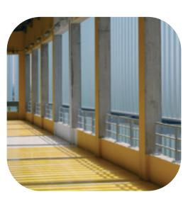
Naturally lit and ventilated: vertically gap-fitted Pilkington **Profilit**\* profile structural glass characterises the design and function of the multi-storey car park.
